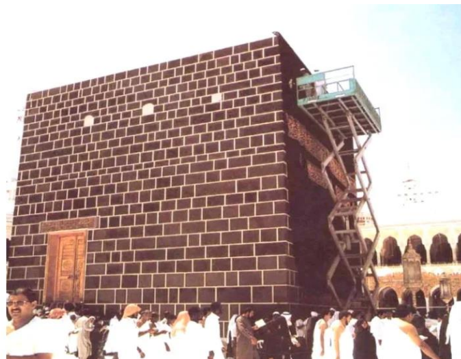
Exposed Kaaba as a New Brocade Covering is being fitted
